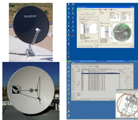
Figure 1. Antenna reception system at the Global Change Unit of the University of Valencia: MSG-SEVIRI reception system (top) and MODIS reception system (bottom).
