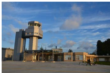
Figure 4. Control tower and auxiliary buildings in Research Center airborne Rozas - CIAR Castro de Rei, Lugo
